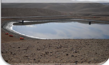
Kidron Facility for Wastewater Treatment
