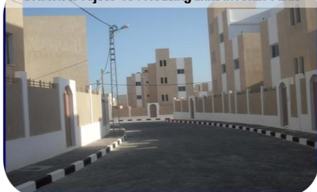
UNRWA Project- 151 Housing units in Khan Yunis
